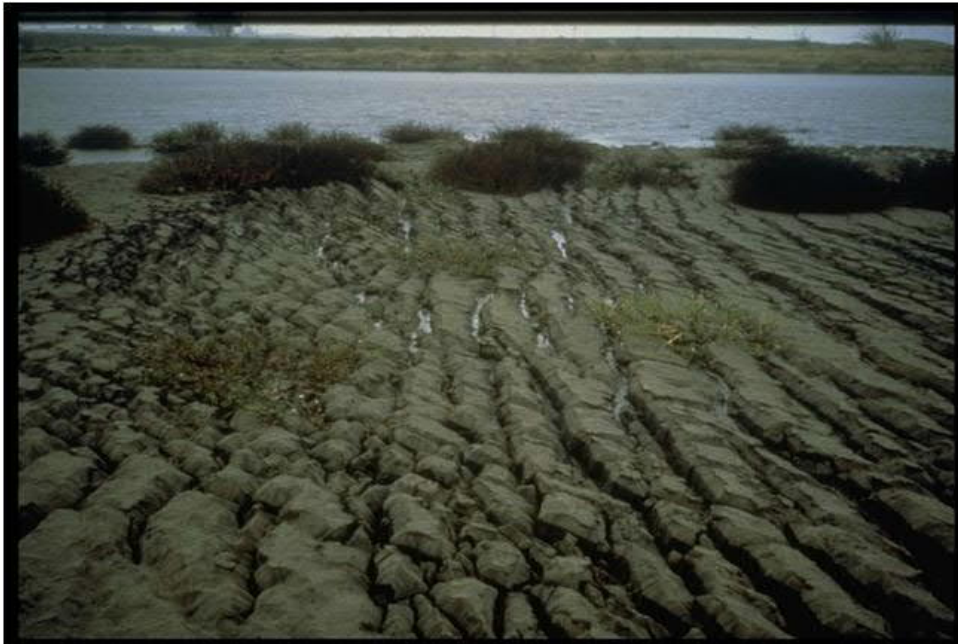
Loma Prieta, California, 1989 - M=7.1
